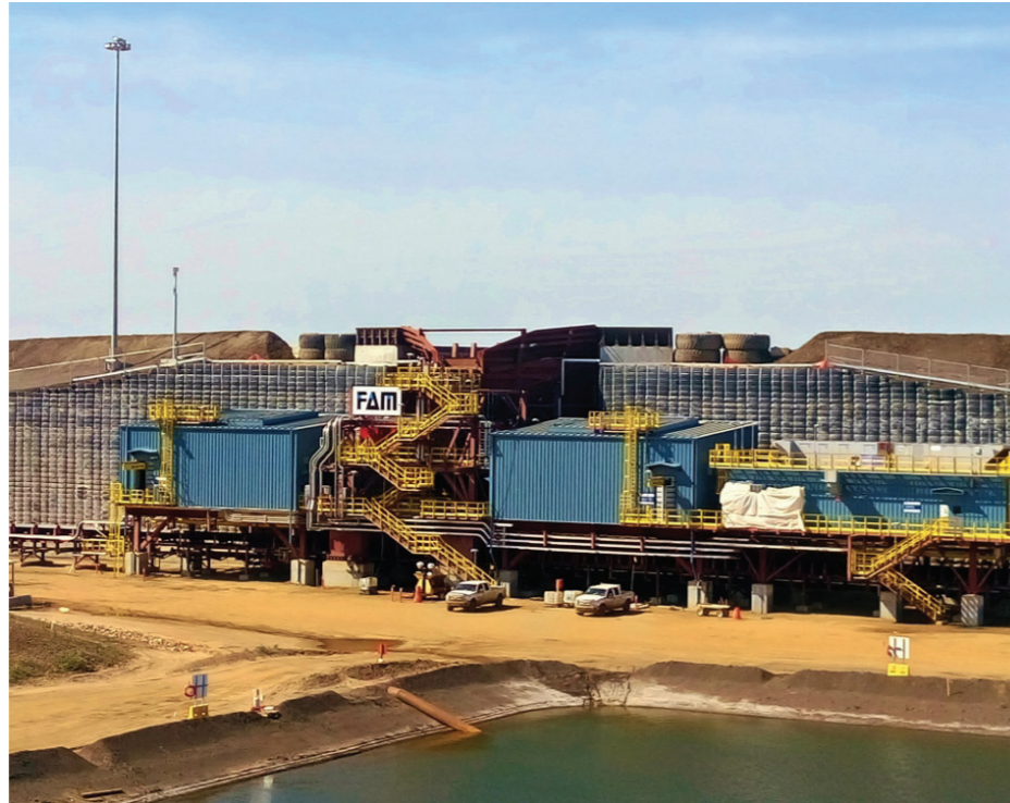
Crushing plant, 2x apron feeder AF3900x21, oil sand 11000 t/h
