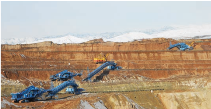
In-pit crushing plant, overburden 5250 t/h, Uzbekistan
