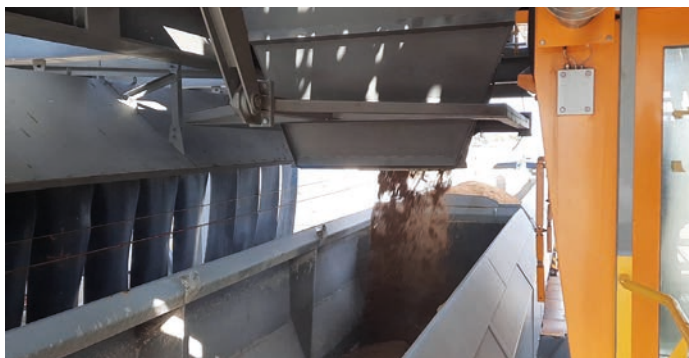
Train loading, lignite 400 - 7500 t/h, Germany
